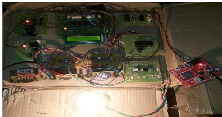
Fig.13: Sending Message of Over Current Providing System By Using the 100w Lamp.
